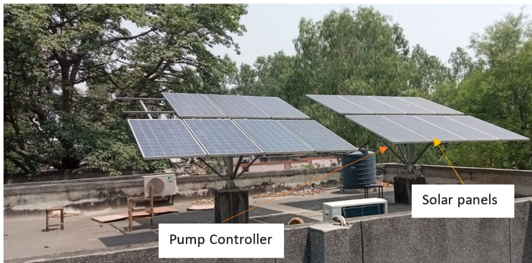
FIGURE 3 Schematic diagram of the solar photovoltaic pumping system.
